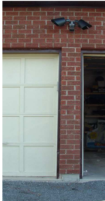
As seen from a 2 meter tall vantage point, the bulbs are not visible at all yet will light up the garage door entry point and the front door walkway
