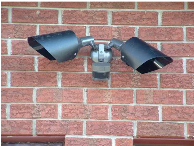
Both shields were attached and some minor adjustments of the light aim and some trimming of the plastic gave us our final product
